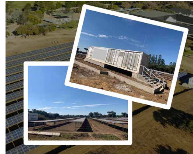
Zimbabwe, 1.5MWh, LFP, Mircogrid
