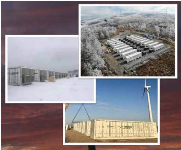
West Virginia, USA, 54MWh, LFP, Frequency Regulation
